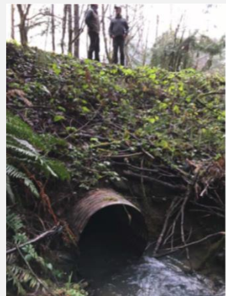
Road Crossing Fish Barrier #1 – downstream view of culvert inlet, Note: This culvert was documented as perched, with and approximate 5 foot plunge below and a complete barrier (PWA, 2010).
